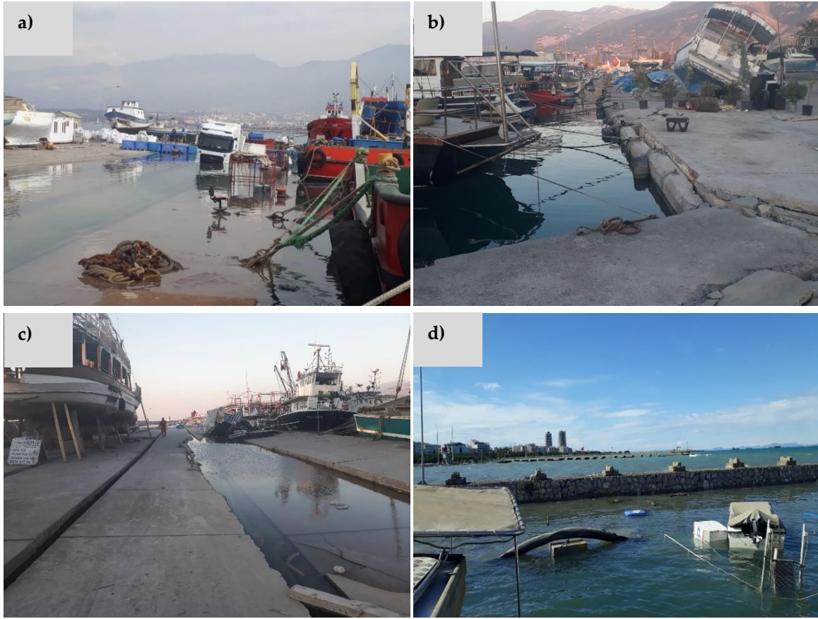
Figure 2. The first images from the Iskenderun Fishing Port after the Kahramanmaraş-epicentered earthquake dated February 7, 2023 (A; The state of the dock at the end of the port, B; The situation of the dock in the middle of the port, C: The collapse of the dock in the middle of the port, D: The collapse at the breakwater level in the middle of the port)
