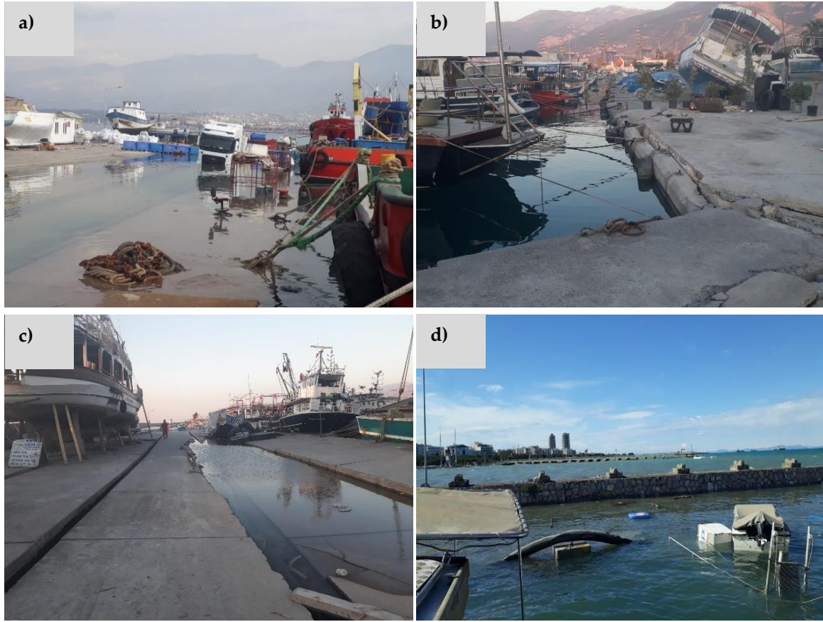
Figure 2. The first images from the Iskenderun Fishing Port after the Kahramanmaraş-epicentered earthquake dated February 7, 2023 (A; The state of the dock at the end of the port, B; The situation of the dock in the middle of the port, C: The collapse of the dock in the middle of the port, D: The collapse at the breakwater level in the middle of the port)
